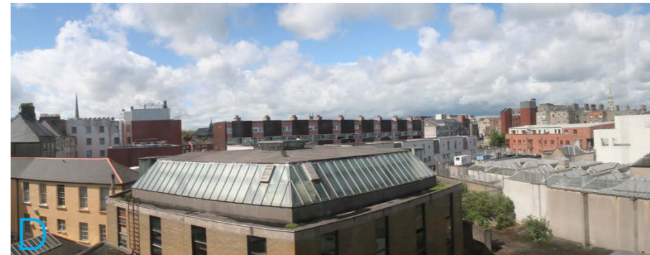
Panoramic View Of Rear Site Looking North
