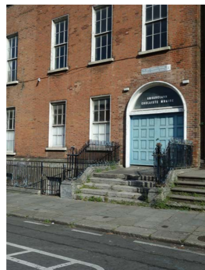
Existing Enlarged Doorway To House 27
