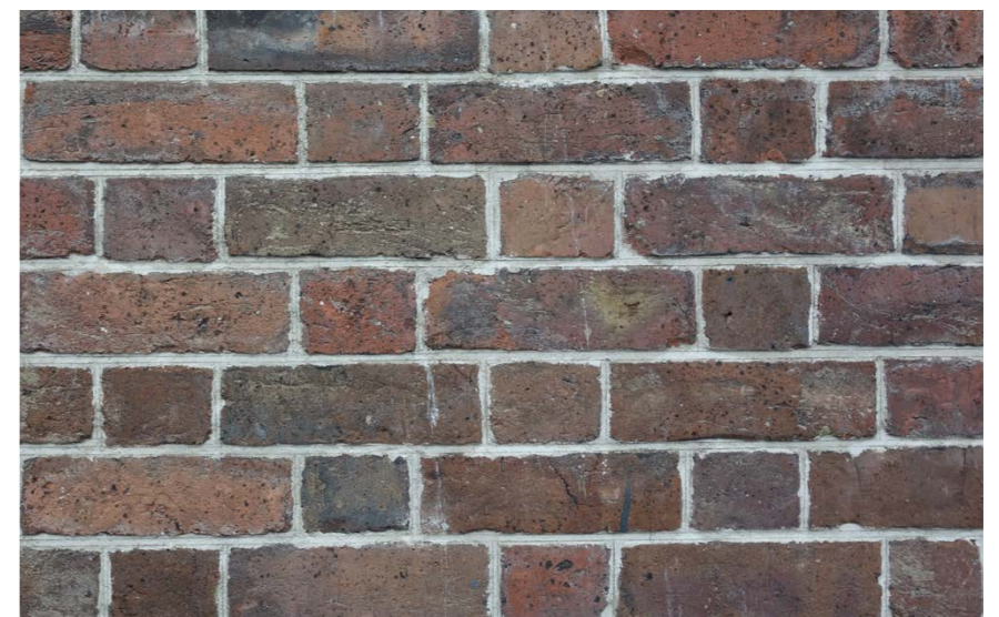
Material Reference: Brickwork
