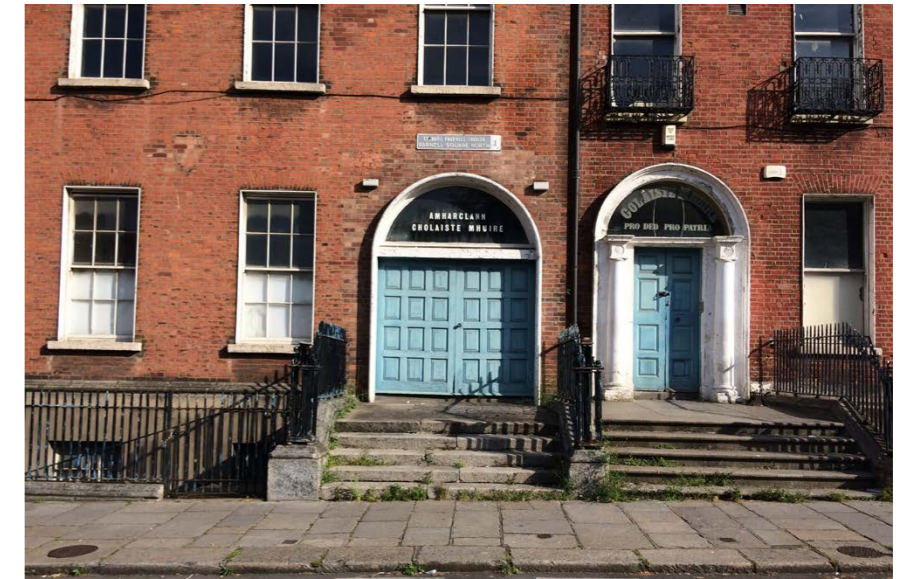
The Stepped Entrances To House Nos 26 & 27
