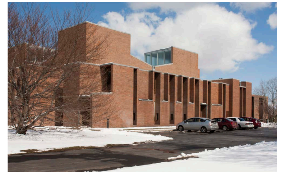
Reference For Restrained Brick Enclosure: First Unitarian Church, Louis Kahn
